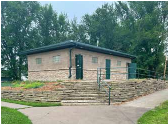
Existing restroom facility at Beach Park
