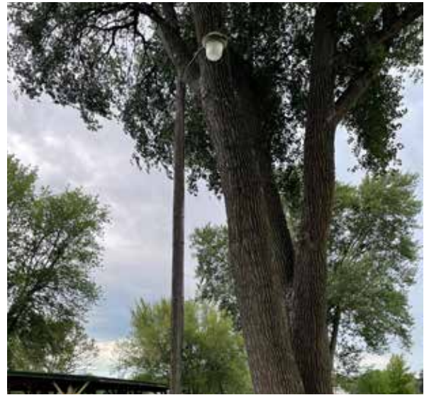
Existing light pole (Convert lighting to LED)
