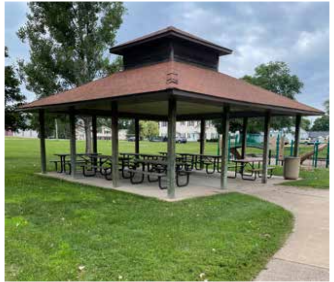
Existing picnic shelter
