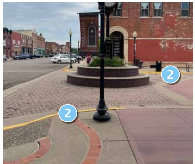
Pavers and ADA accessibility issues near clock tower
