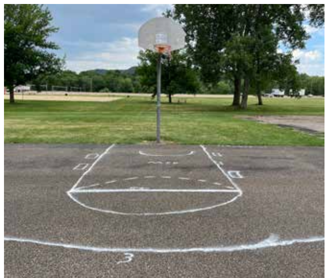
Existing basketball court
