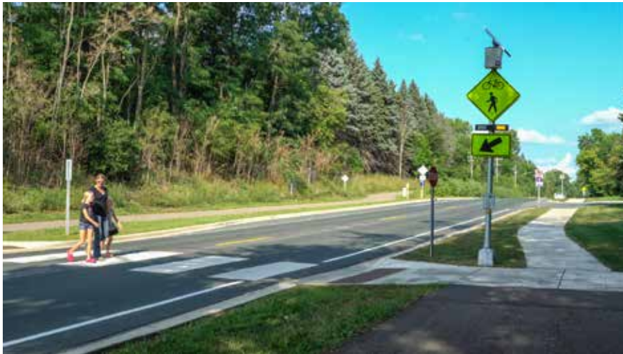
Proposed crossing treatment: This example from West Saint Paul shows an RRFB system and high visibility crosswalk demarcations providing drivers with clear indications of potential pedestrian activity.
