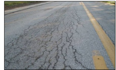
Pavement Cracks
