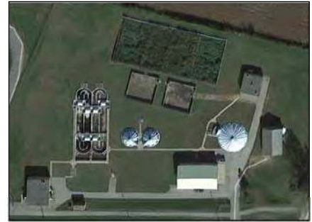
Wabasha Wastewater Treatment Plant
