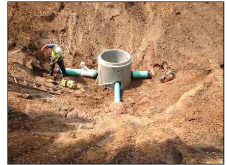
Shields Avenue Manhole
