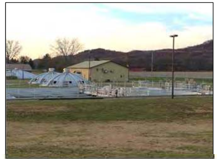
Wabasha Wastewater Treatment Plant
