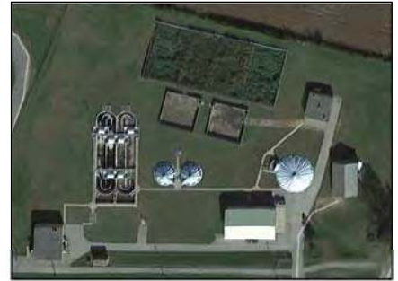
Wabasha Wastewater Treatment Plant
