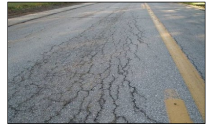
Pavement Cracks
