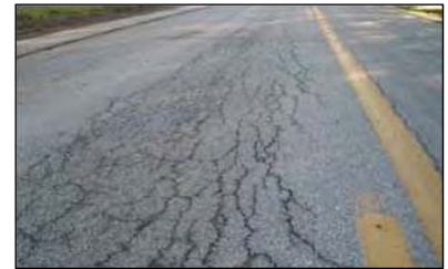
Pavement Cracks
