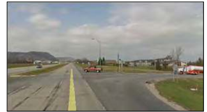
Highway 61, Principal Arterial
