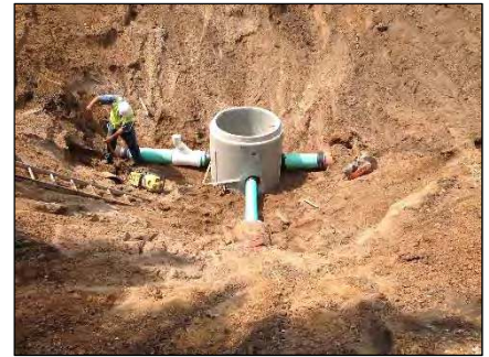
Shields Avenue Manhole
