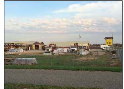
Interstate Building Supply
