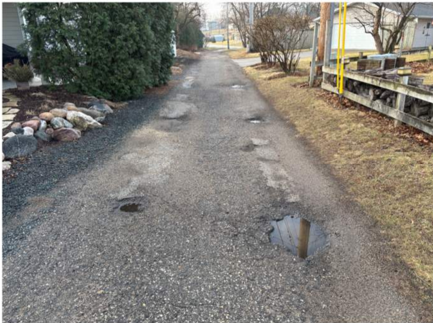
Alley mid-block between Lawrence Boulevard East and Main Street East looking south
