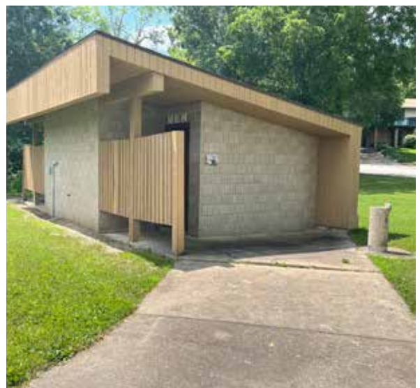
Restroom facilities (Update)
