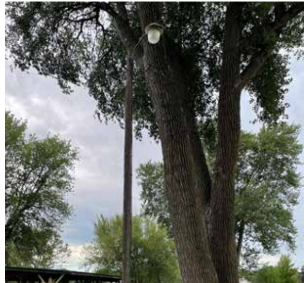
Existing light pole (Convert lighting to LED)
