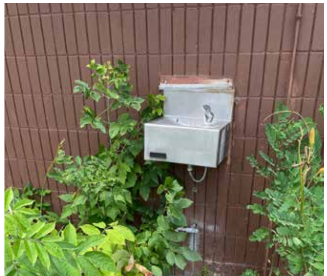
Existing drinking fountain
