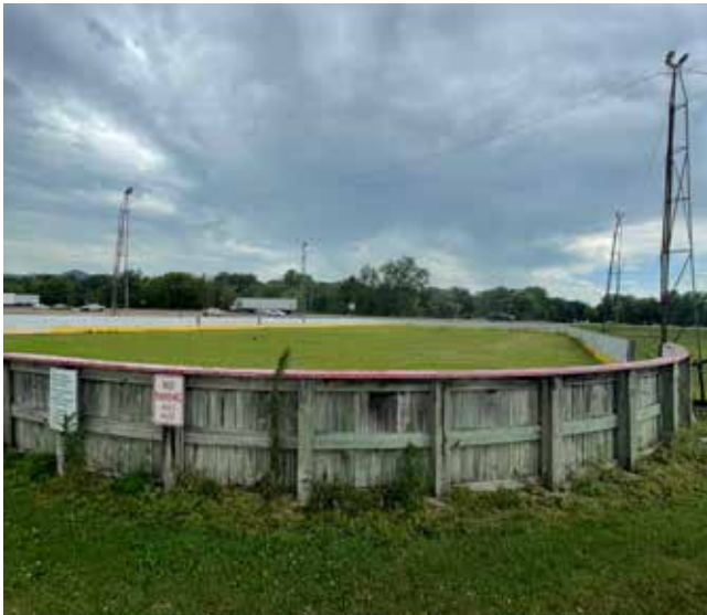
Existing enclosed hockey rink area
