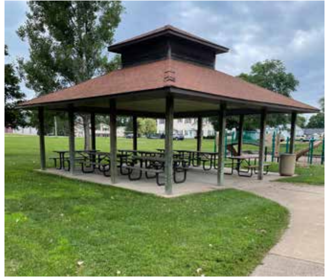
Existing picnic shelter
